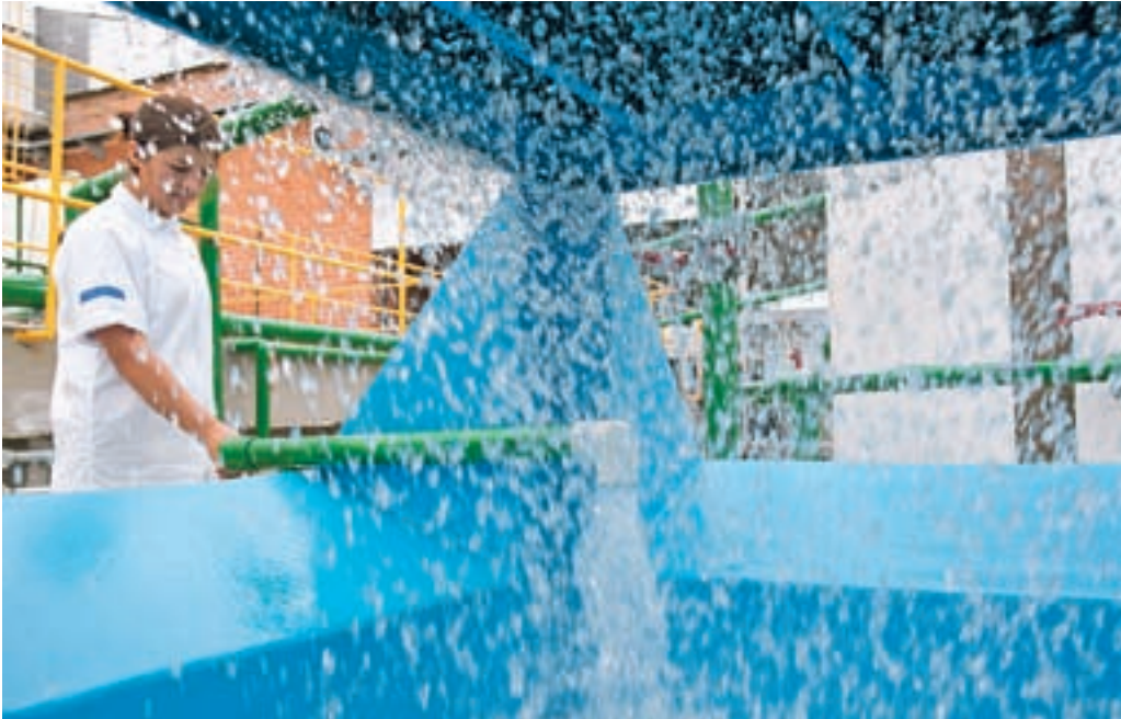
The Alimentos Cárnicos drinking – water treatment plant; La Ceja, Colombia.
