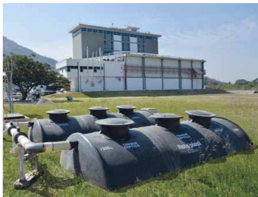
The wastewater – treatment plant, Molino Santa Marta ; Santa Marta, Colombia.
