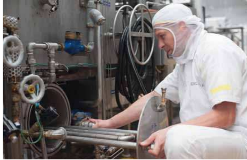
Heating coils in the demolding tank, Meals de Colombia Plant; Bogotá, Colombia.
